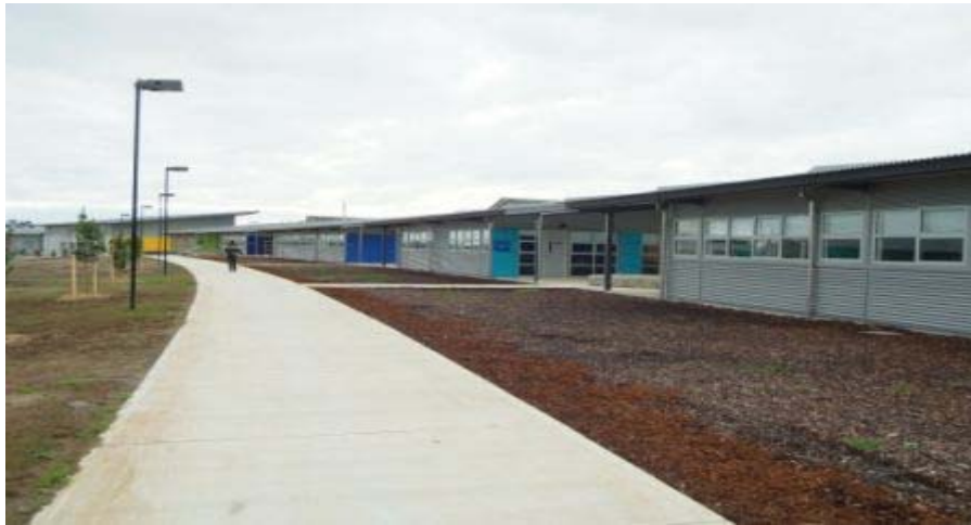
Above: Auckland Region Women's Corrections Facility
